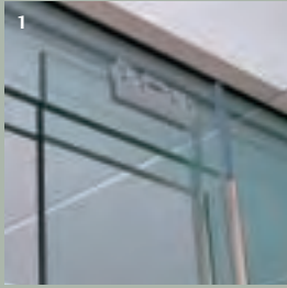
1 Sliding door in double glazed at head
